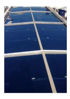
Providing outstanding resistance to extreme weather conditions, Avery Dennison R SkyLite 20 XTRM Poly solar control exterior window film is designed for application on flat, curved and sloped roofing systems.
