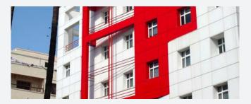
**Façade Film** This premium cast film is perfect for panels, window frames for restoration, restyling or branding purposes. Its high adhesion onto difficult building substrates such as plastics, aluminium, steel and reinforced facade panels makes it an excellent alternative to paint. Comes with a life expectancy of up to 7 years.
